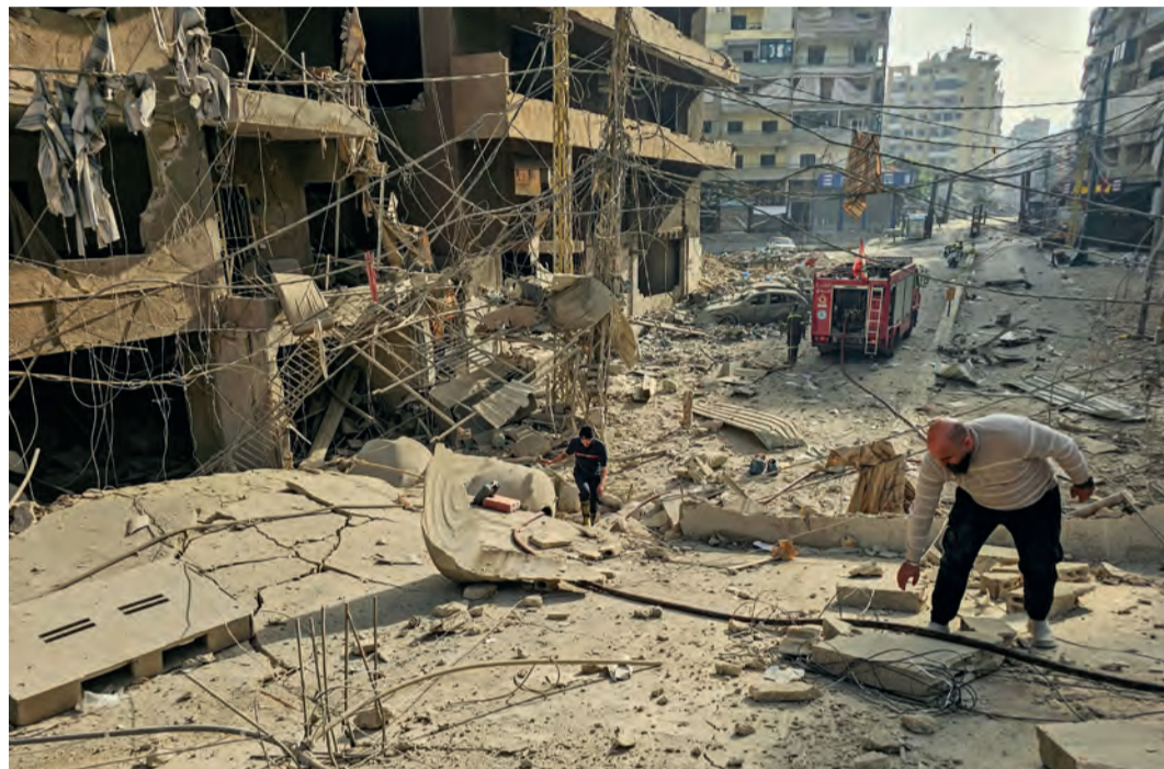
A man stands on the rubble of a destroyed building as firefighters work at the site of overnight Israeli airstrikes in the Haret Hreik neighbourhood of Beirut's southern suburbs
